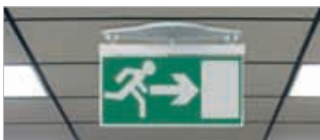
Surface Exit Sign
